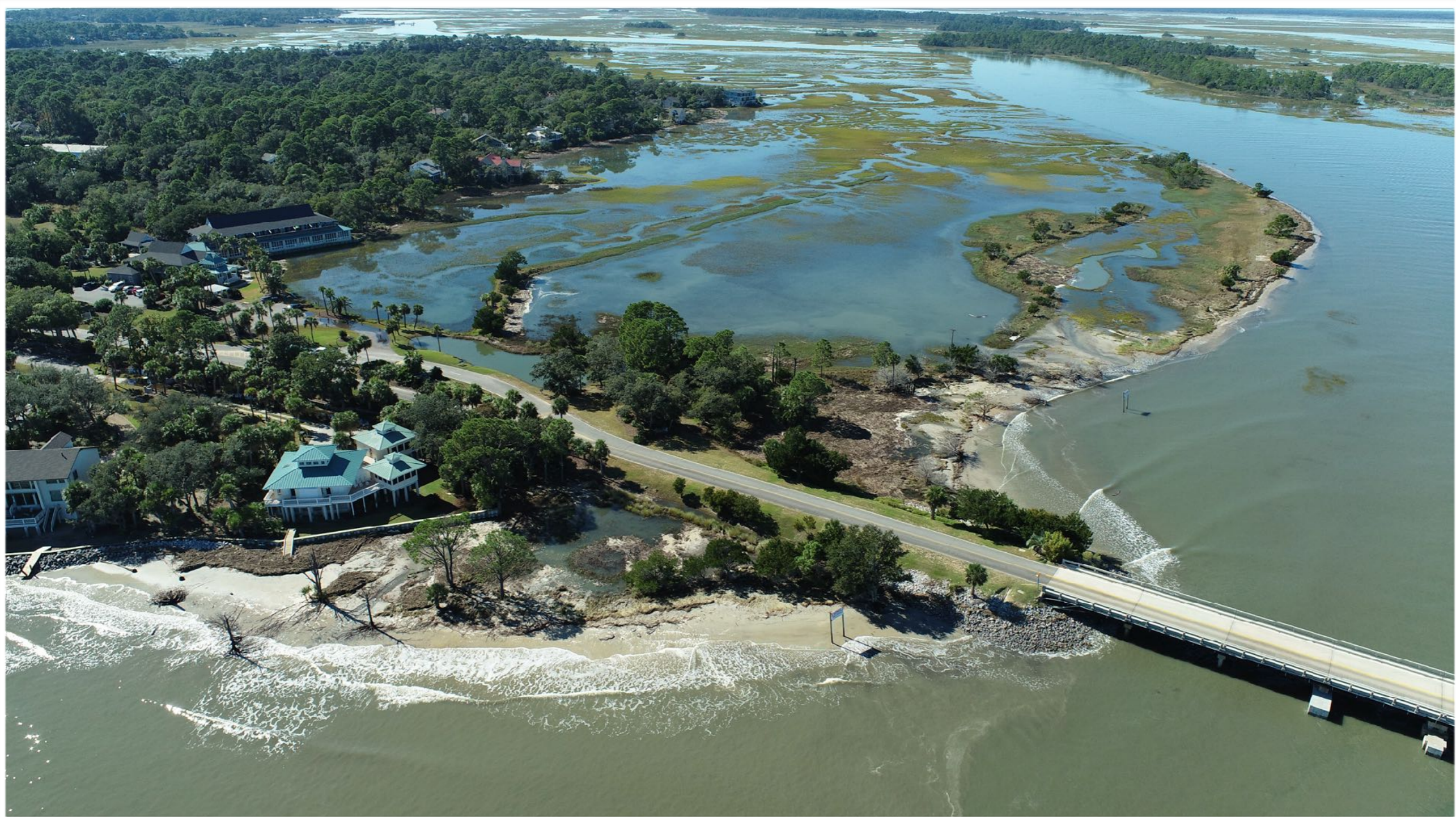
Fripp bridge abutment.
