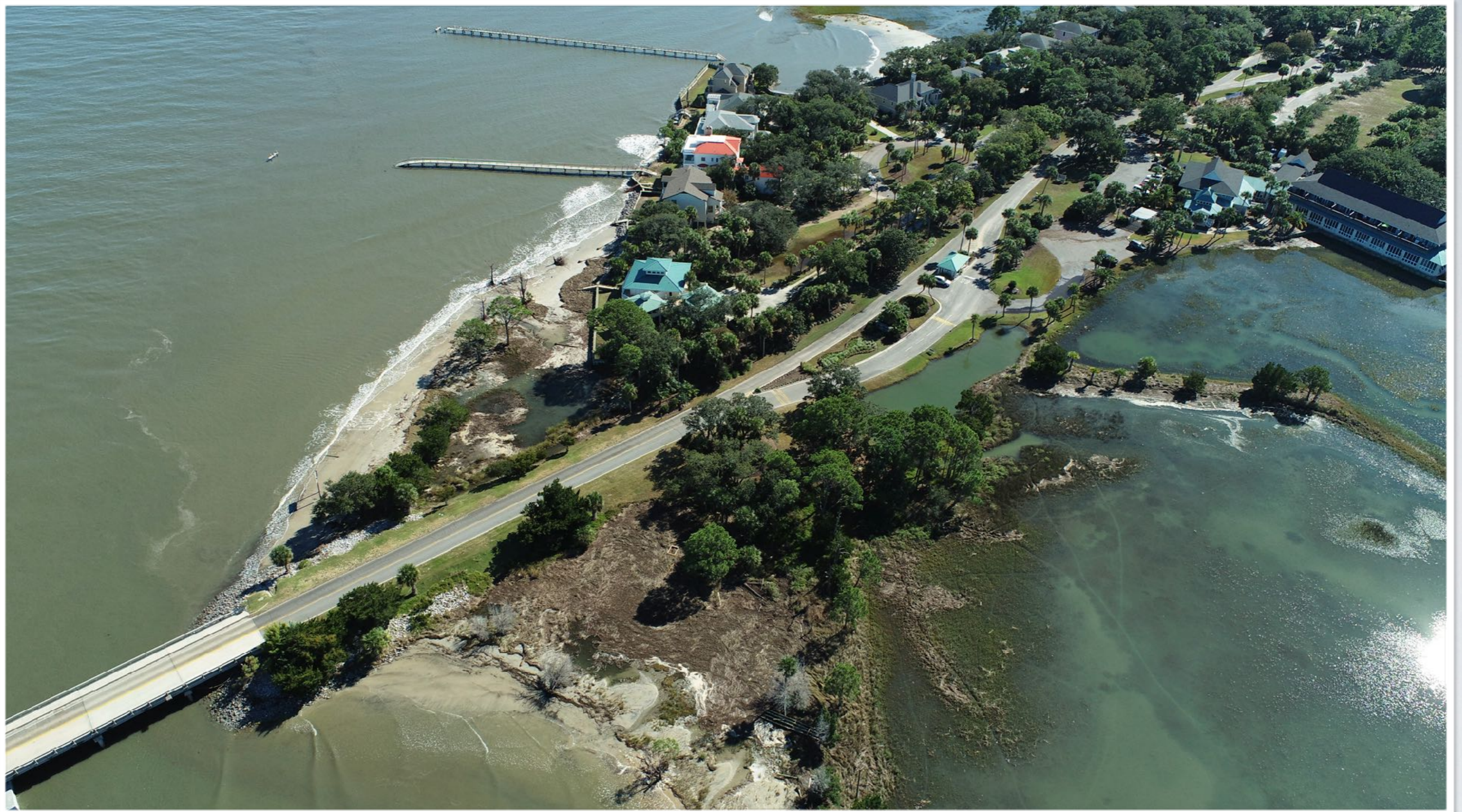
Fripp bridge abutment.
