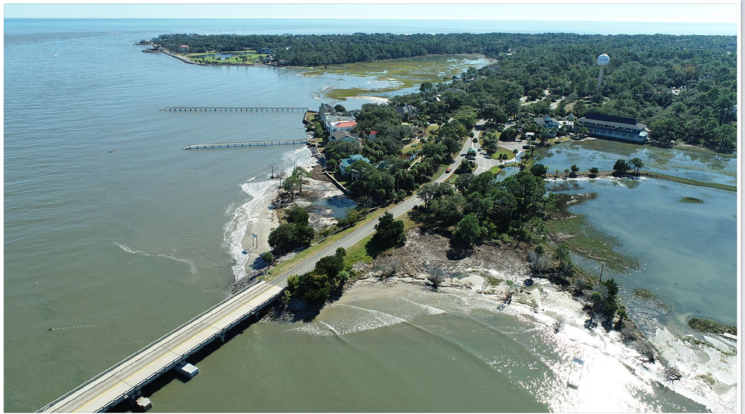
Fripp bridge abutment.
