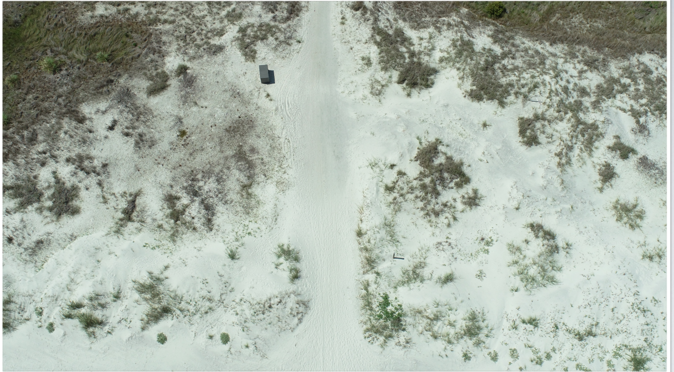
Access # 15. Closeup view. New sand dunes are forming at the end of the geo-webbing expanding the distance from the end of the access to the beach.
