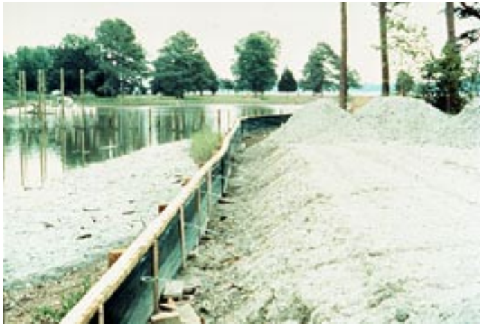
Figure 11. Note the filter cloth lining the landward face of this bulkhead.
