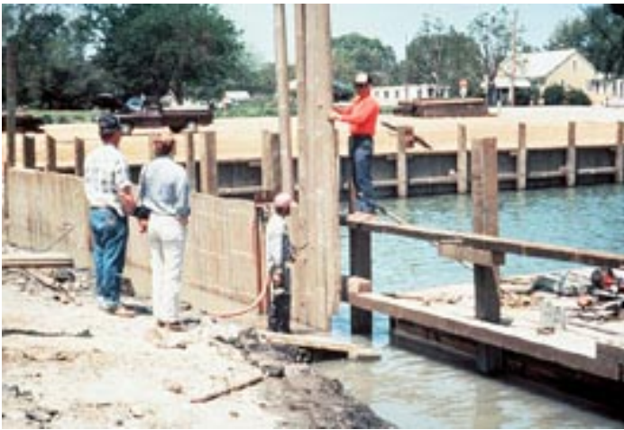
Figure 6. Installing sheet piles.
