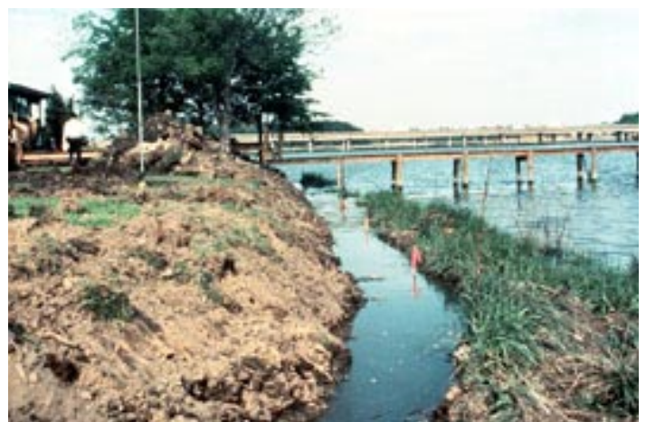
Figure 22. Toe of riprap revetment/landward of fringe marsh.
