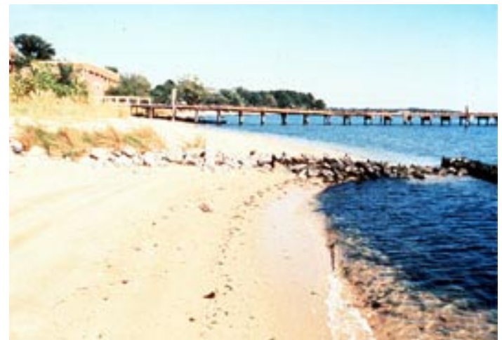
Figure 49. Riprap groin trapping sand.
