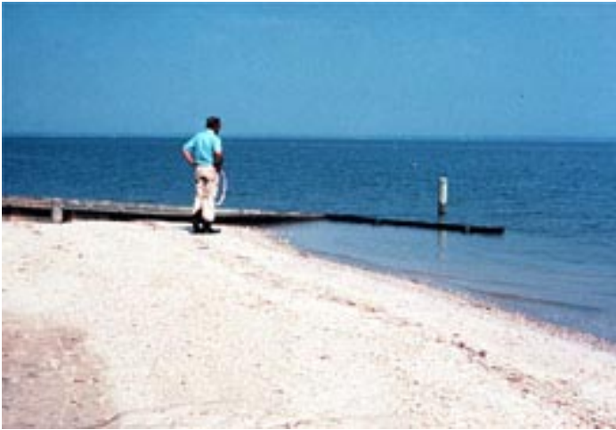
Figure 46. Groin with spur.
