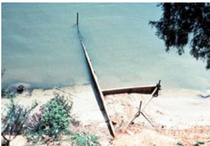
Figure 54. Spur prevents erosion on downdrift side of groin.
