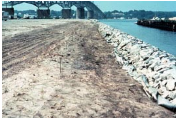
Figure 58. Riprap protecting a channel.
