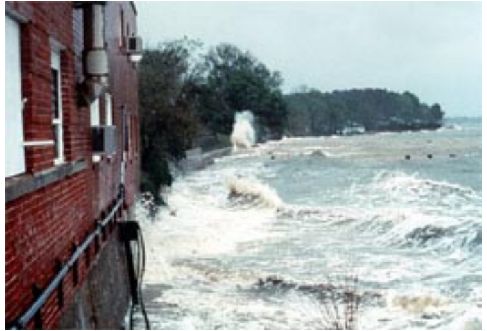
Figure 67. Bulkhead reflecting wave energy.
