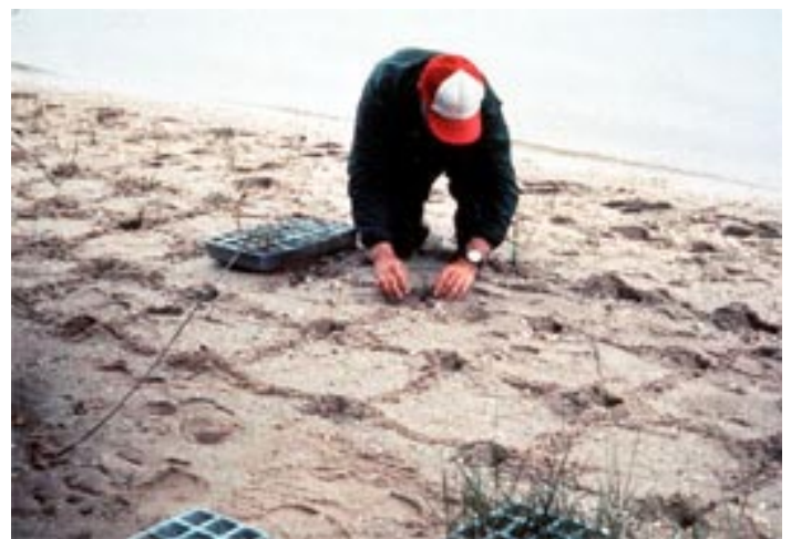
Figure 63. Planting on 18" center grid.
