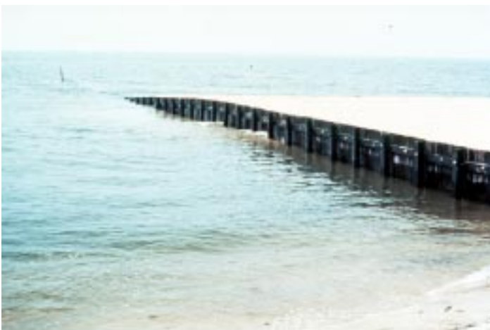
Figure 44. Groin trapping sand on updrift side.
