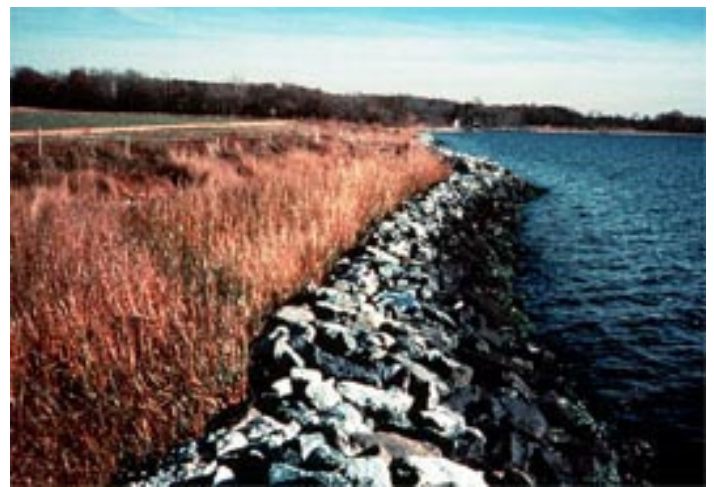
Figure 25. Revetment provides habitat and erosion protection.
