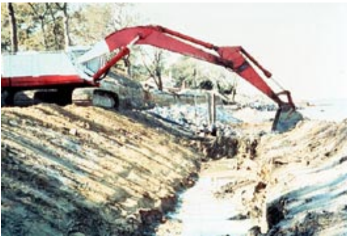
Figure 19. Riprap buried toe construction.
