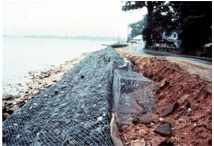
Figure 34. Revetment made of gabion baskets.
