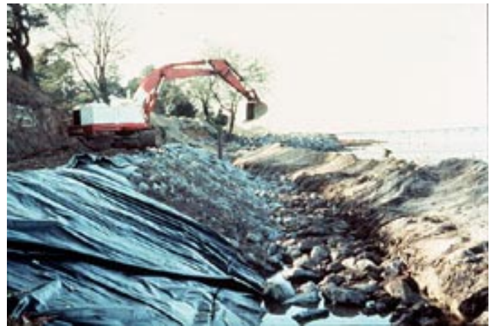
Figure 20. Core stone being placed on filter cloth.
