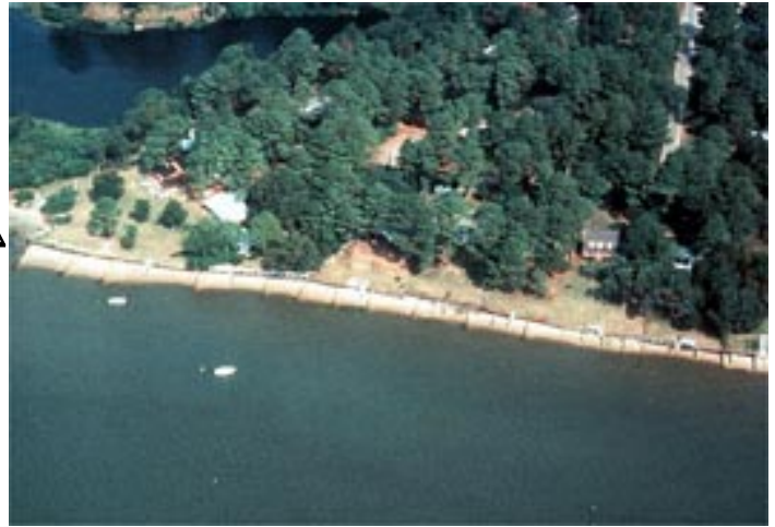
Figure 47. Downdrift erosion at end of groin field.
