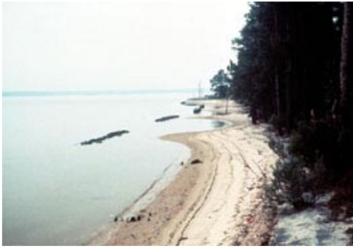
Figure 38. Typical tombolo formation landward of breakwater.
