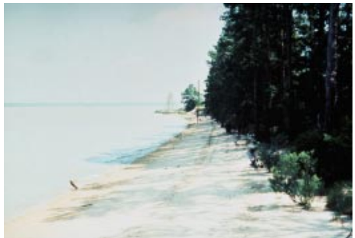
Figure 37. Beach before installation of offshore breakwaters.
