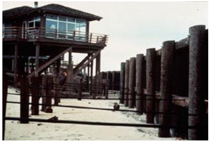
Figure 7. Tie back rods.
