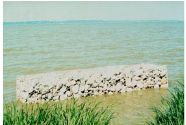
Figure 33. Gabion basket breakwater.
