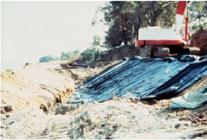
Figure 23. Revetment constructed with filtercloth.
