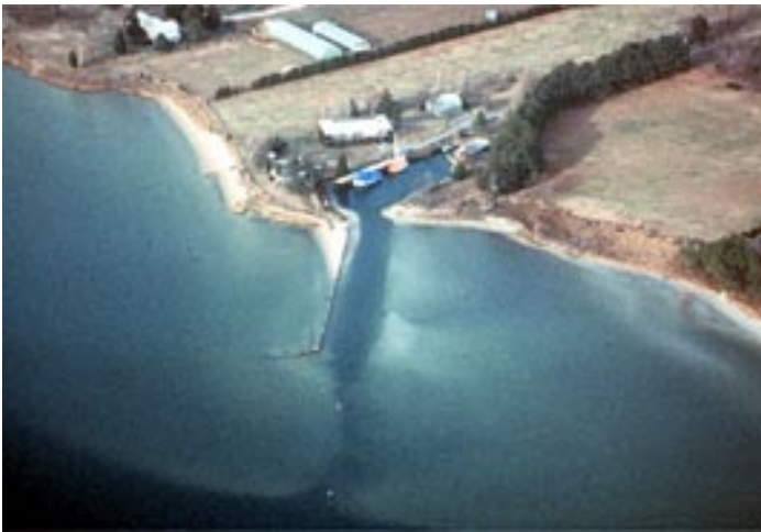
Figure 61. Single jetty protecting channel.
