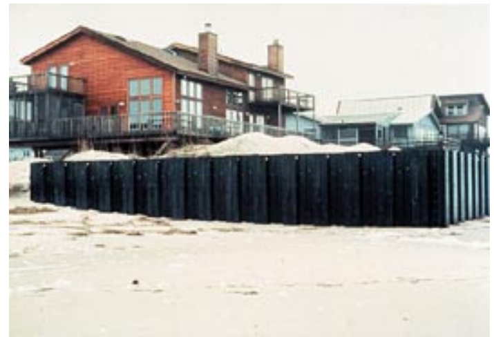
Figure 10. Steel bulkhead (return wall).
