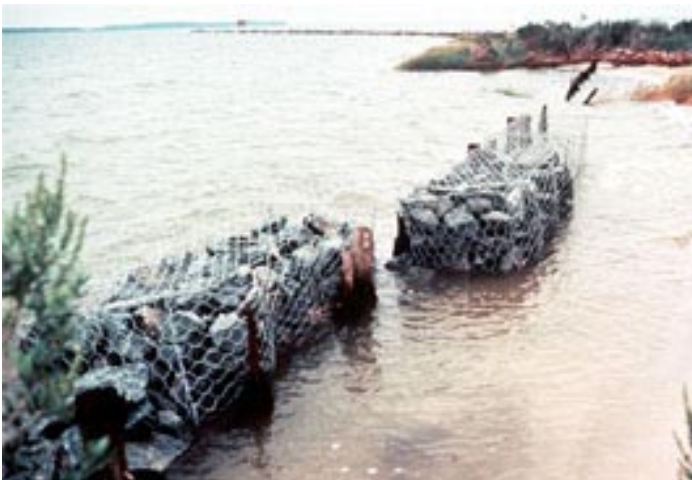
Figure 32. Gabion baskets forming a gapped breakwater.
