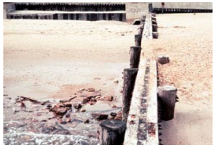
Figure 45. Groin trapping sand.
