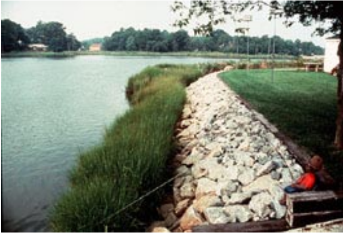
Figure 14. Properly designed riprap revetment.
