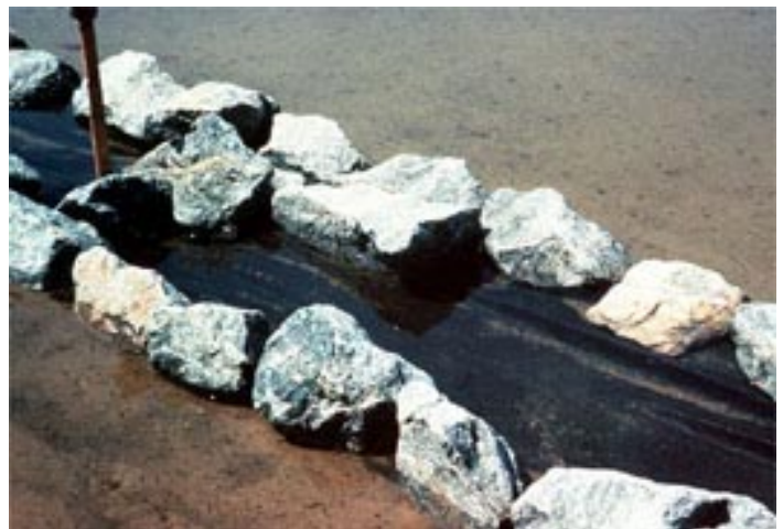
Figure 50. Riprap groin placed on filter cloth.
