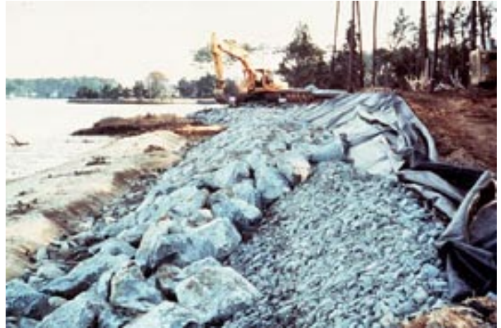
Figure 15. Armor stone set on base of core stone and filter fabric.
