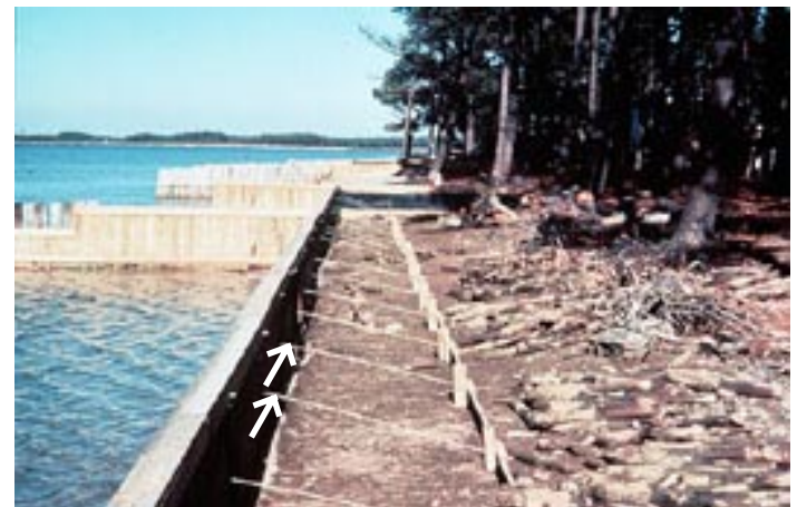
Figure 9. Galvanized rod tie-backs.
