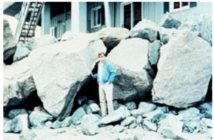
Figure 16. Riprap must be sized for expected wave height.
