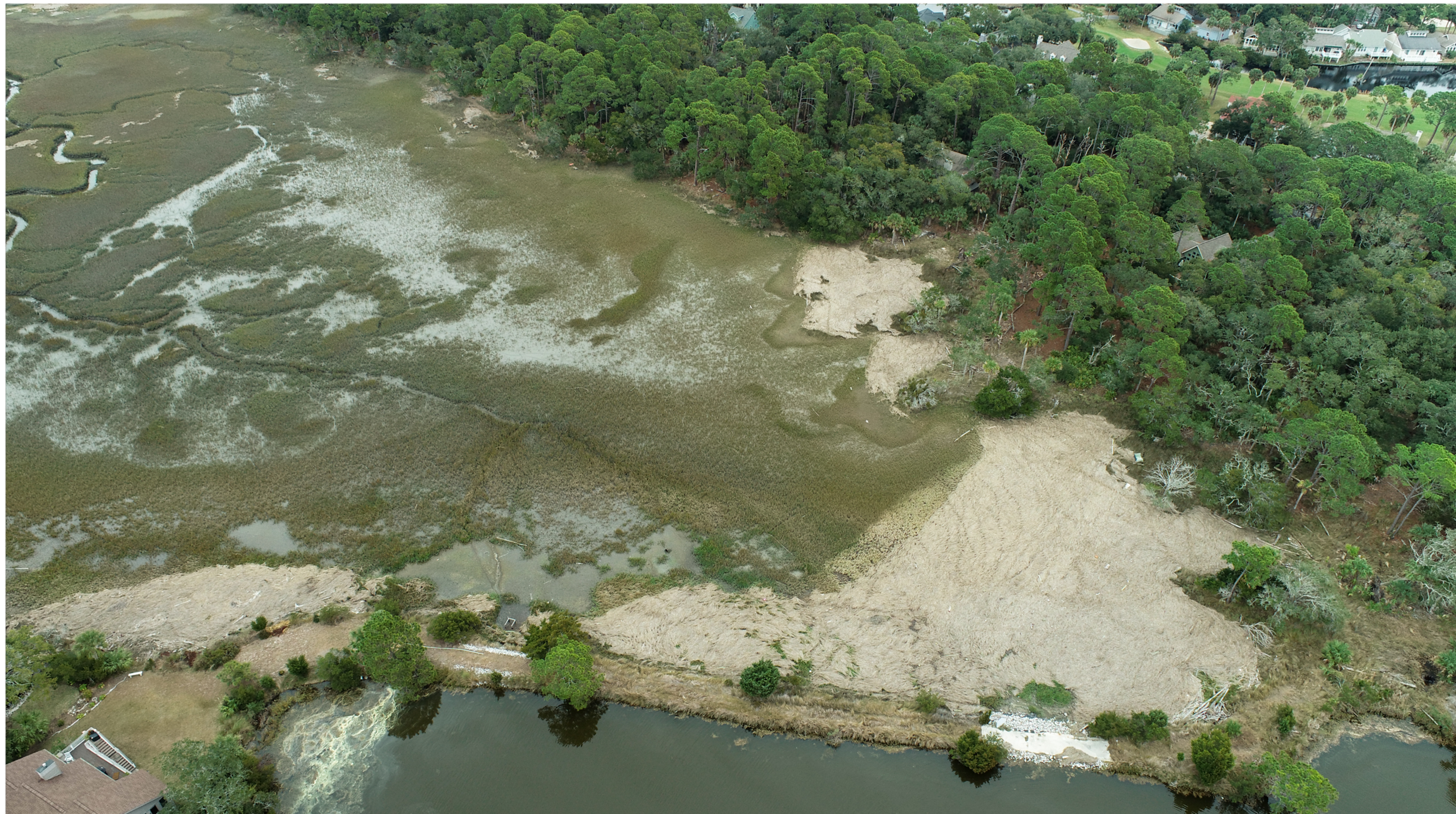
January 21, 2022 - At the end of the salt marsh is a spillway that overflows into Deer/Blue Heron lake. Because the eroded area has expanded so far into the marsh, it leaves huge quantities of wrack piled up at the end of the marsh's boundary during flood events.
