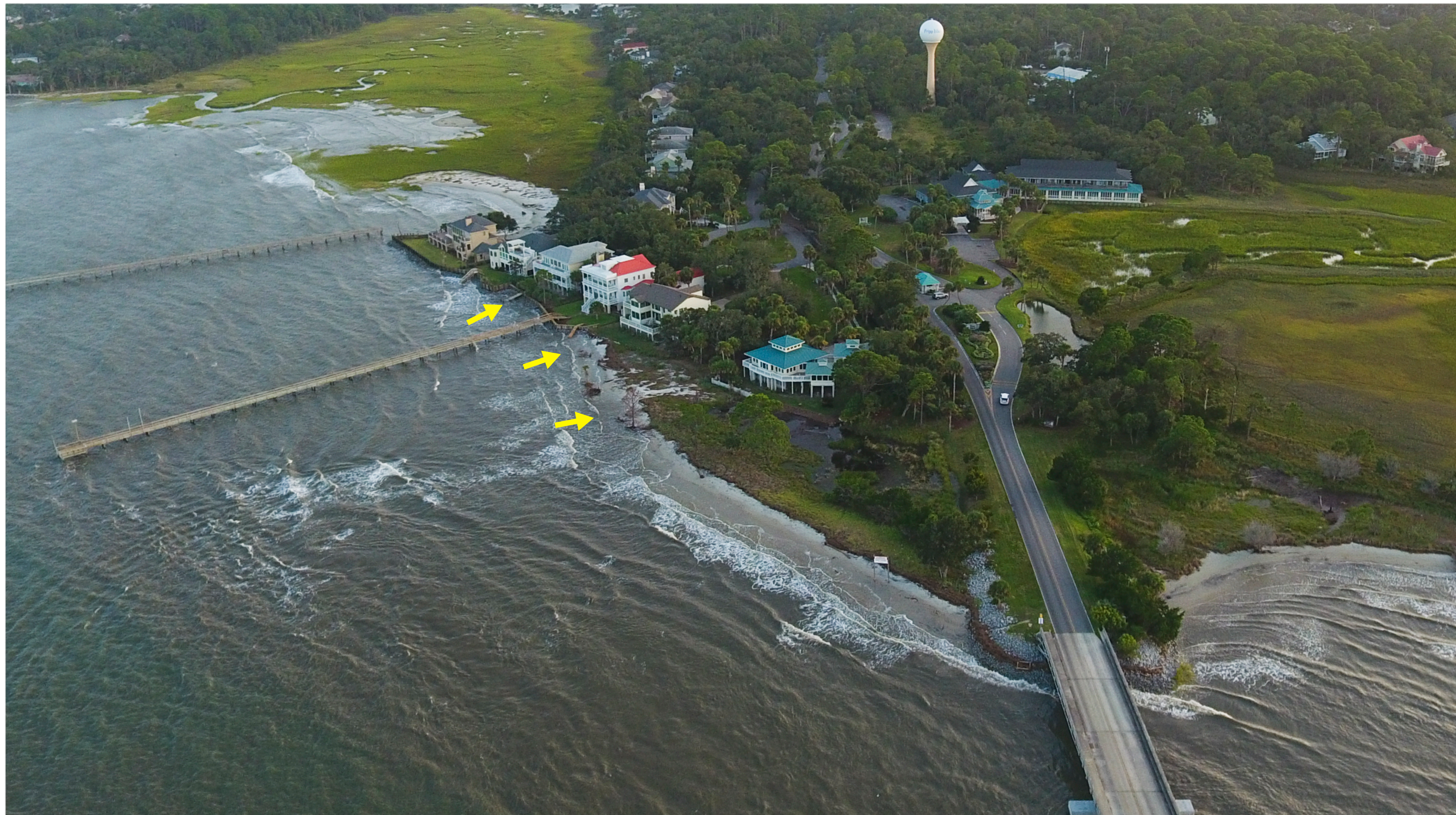
This photo, taken two years later on September 17, 2020 , during a normal high tide, shows the eroded area has expanded along the front of the River Club homes and towards the bridge approach area.
