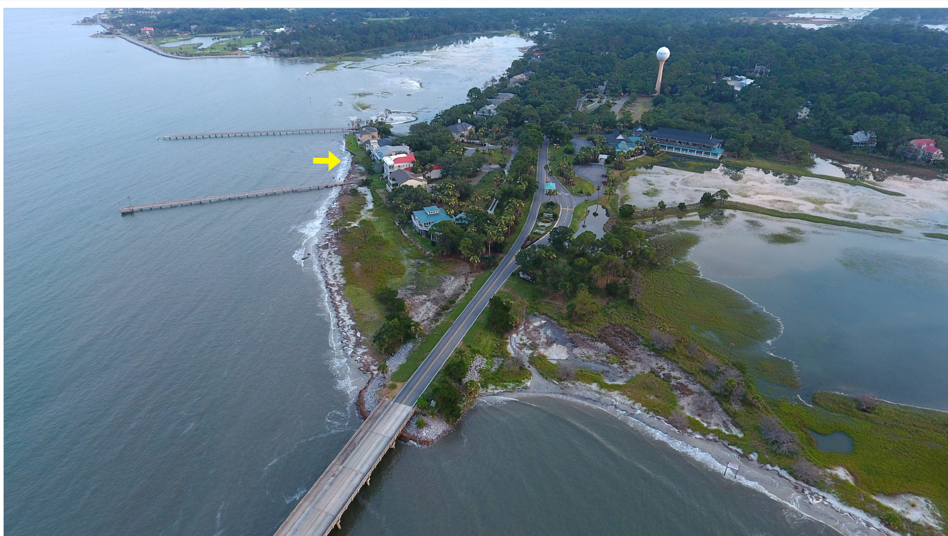
This aerial photo, taken during a king tide event on July 13, 2018 , shows the grassy area in front of the homes remains for-the-most-part, dry and intact even during higher than normal flooding.
