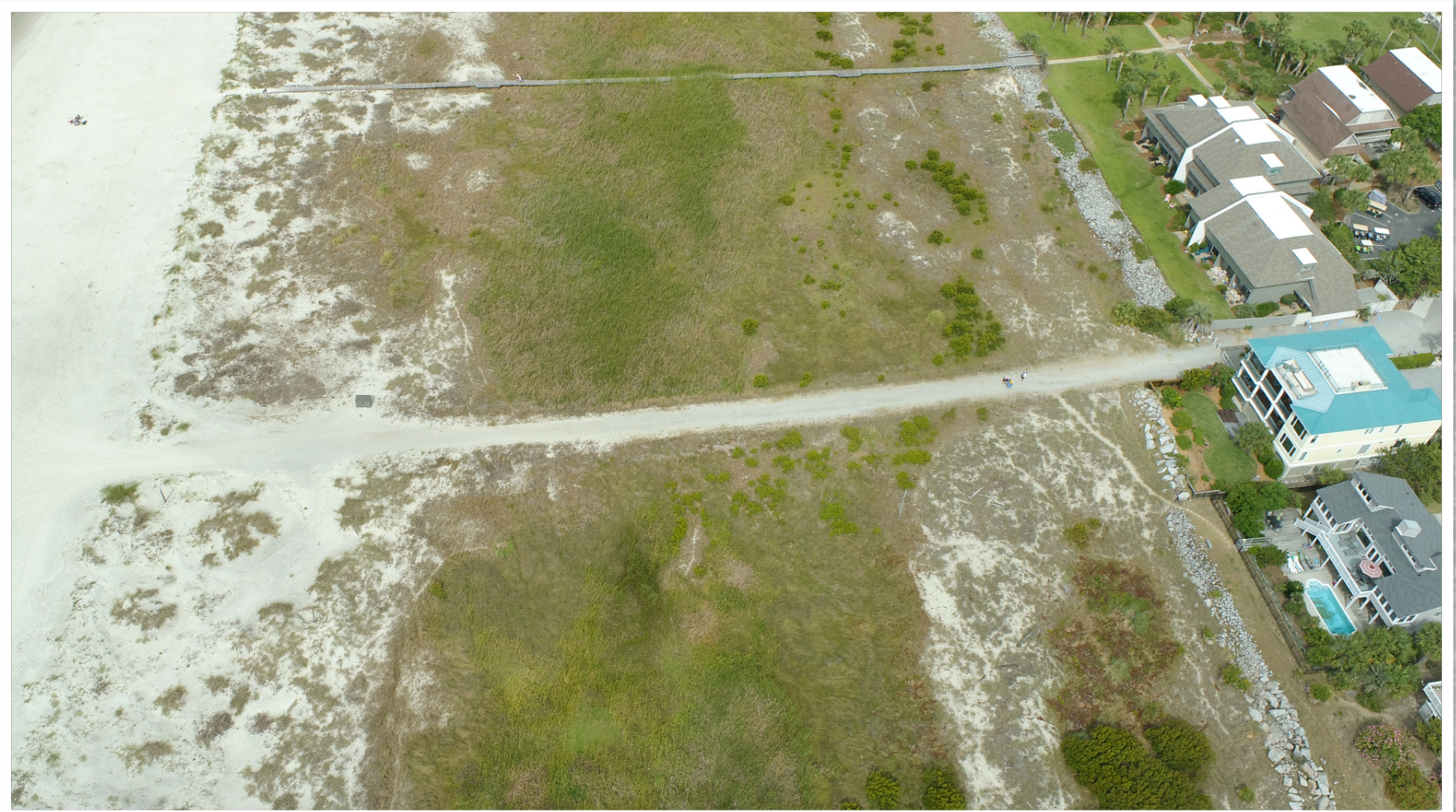
Detail of access #15 - Overall view of the full length of the access.
