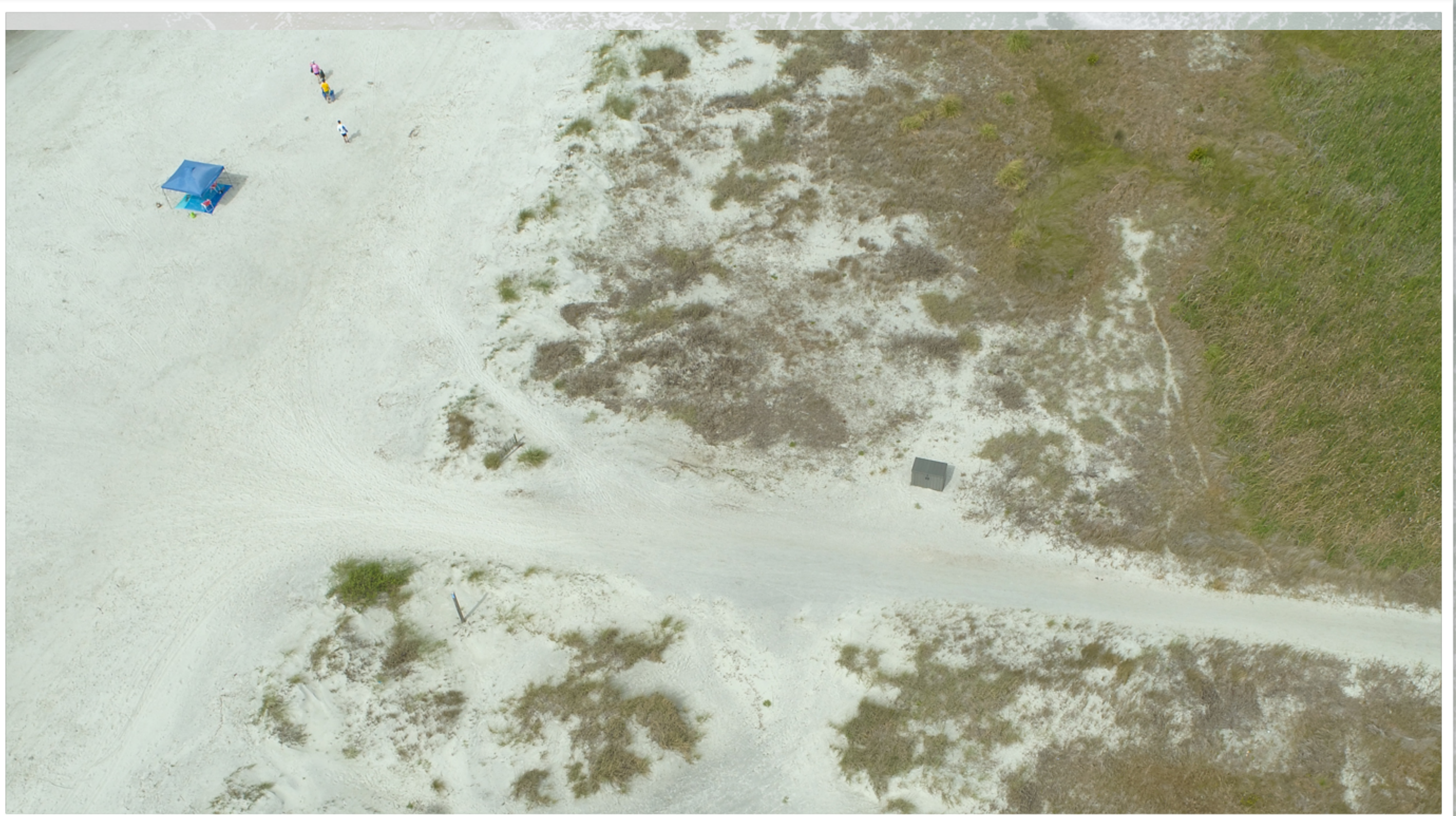
Detail of access #15 - An aerial view of the beach end of the access where traction problems have been occurring with handicap vehicles.
