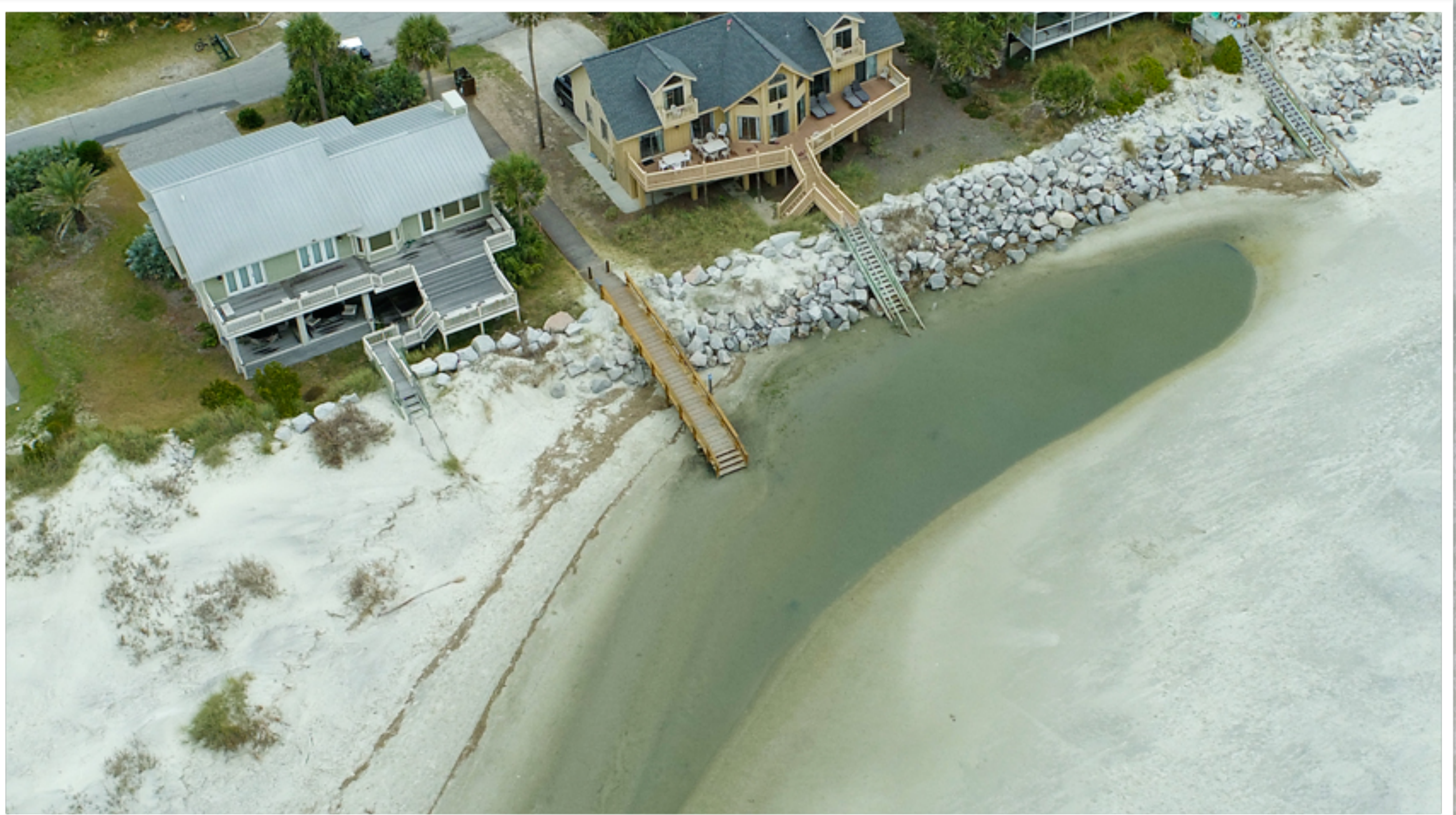
Detail of access #1B - Aerial view of the access walkway taken during low tide. Also visible in this photo is the wrack line from the May 24th king tide at the revetment, as well as a typical high tide wrack line as it relates to the access walkway and stairs.
