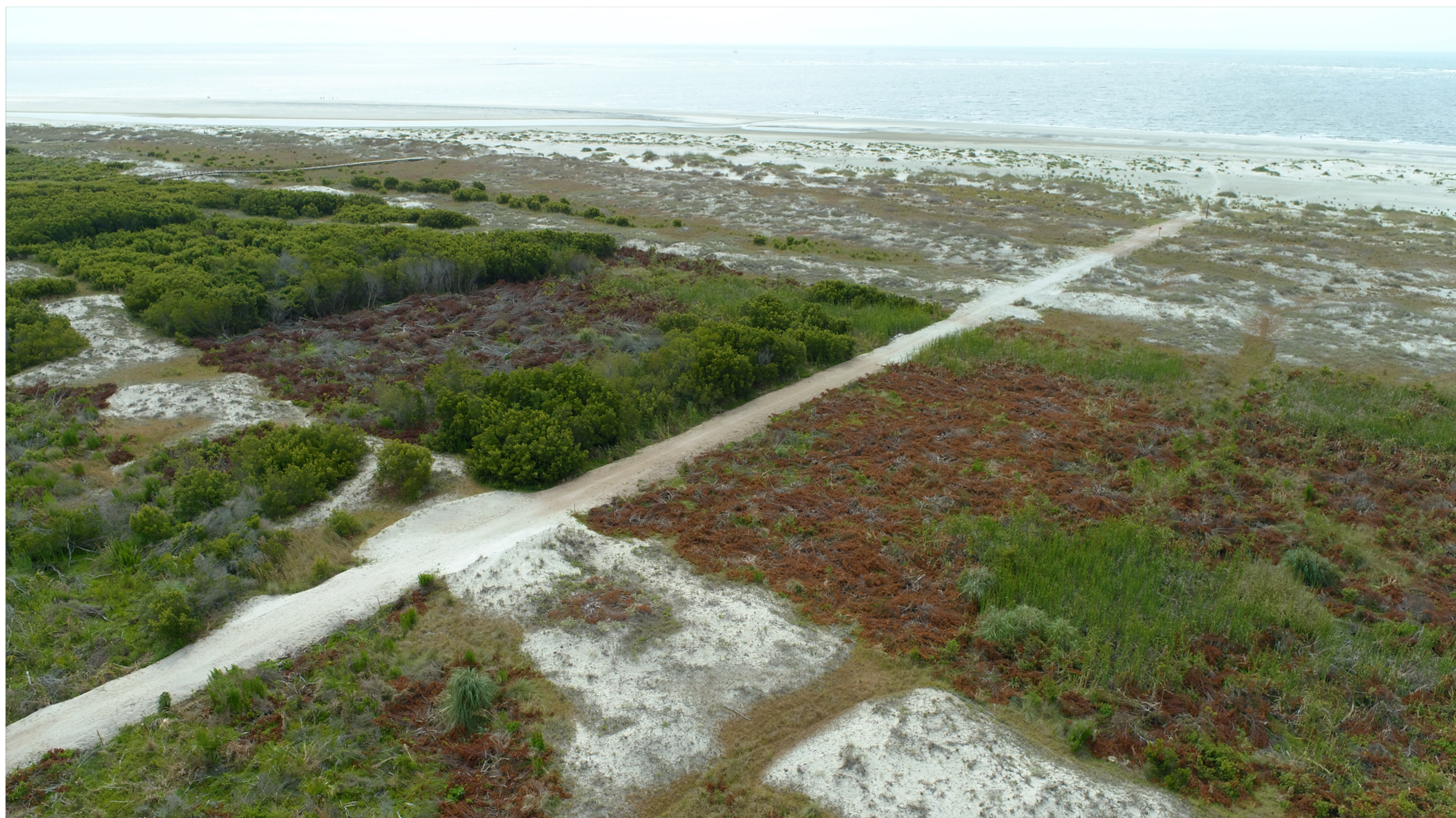
Detail of access #4 - path - level, straight path all the way out to the beach allowing emergency vehicles access to the northern end of the beach.
