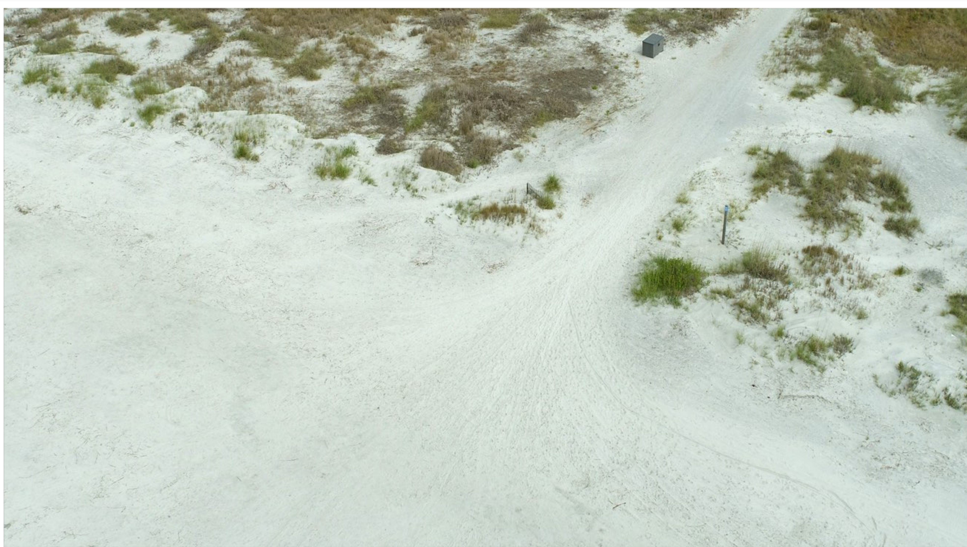
Detail of access #15 - Another view of the area where beach sand meets the access path. This area contains a loose granular surface that can cause traction problems for handicap vehicles.
