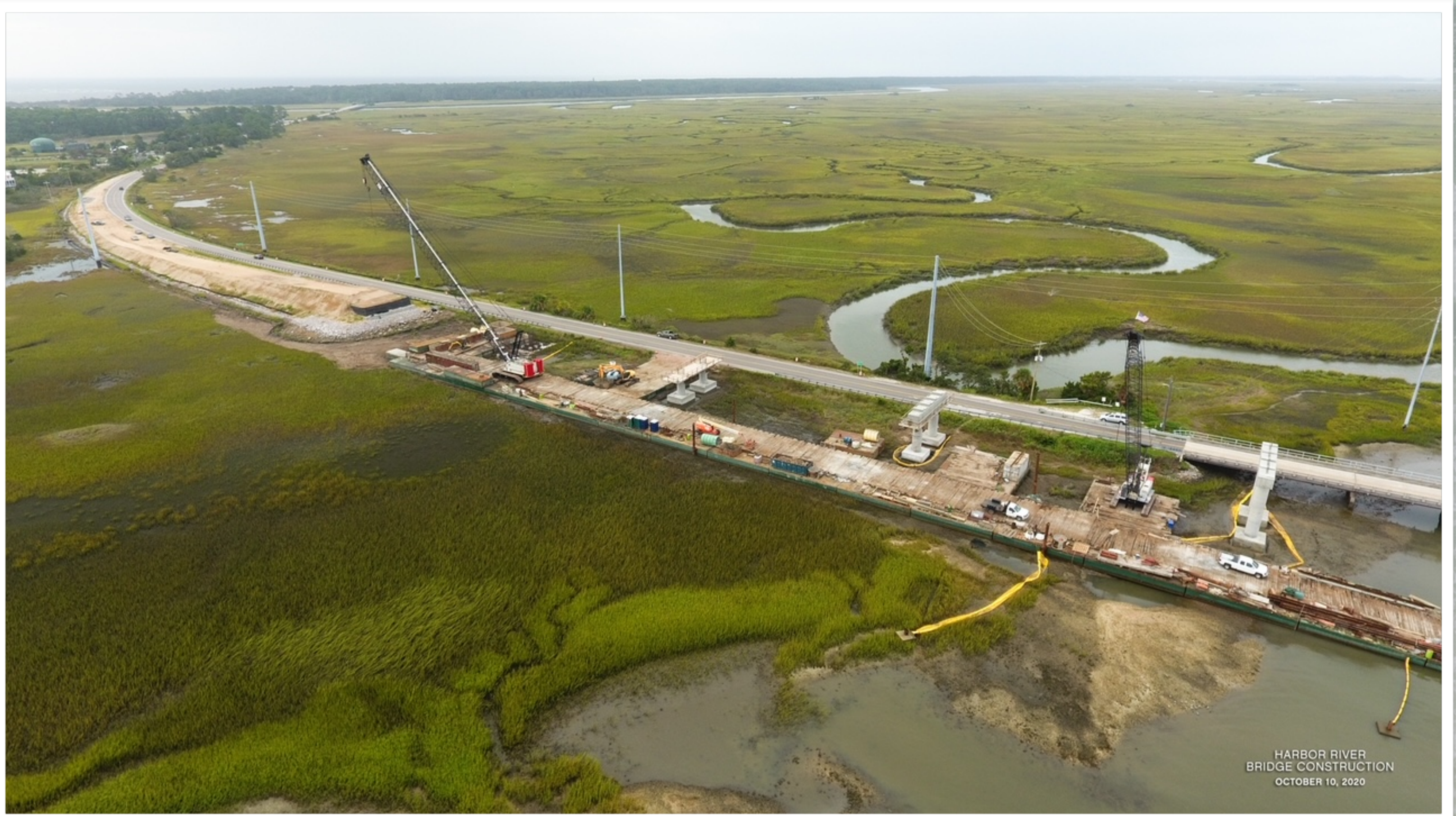
Harbor River bridge under construction
