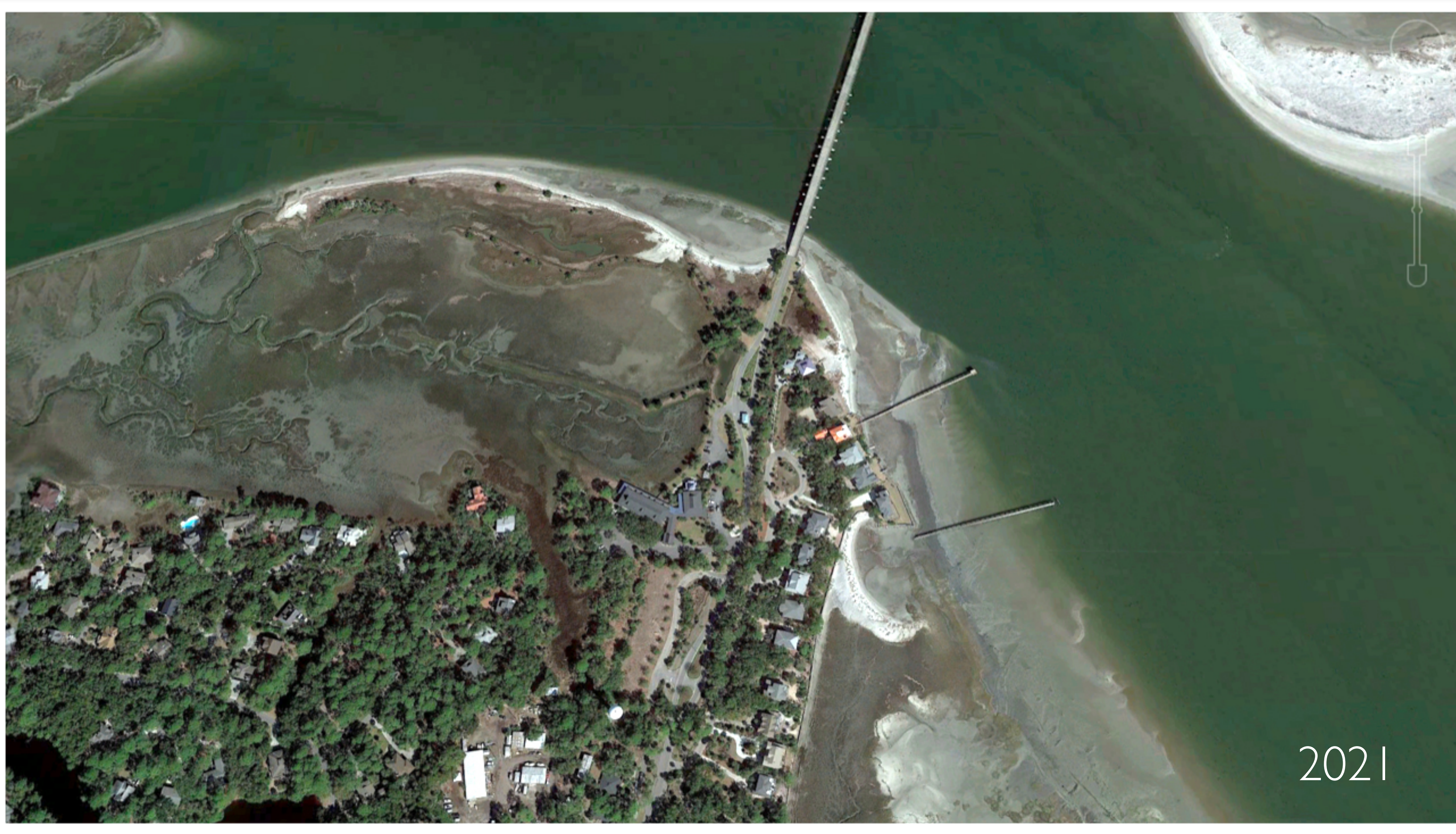
The bridge area of Fripp Island
