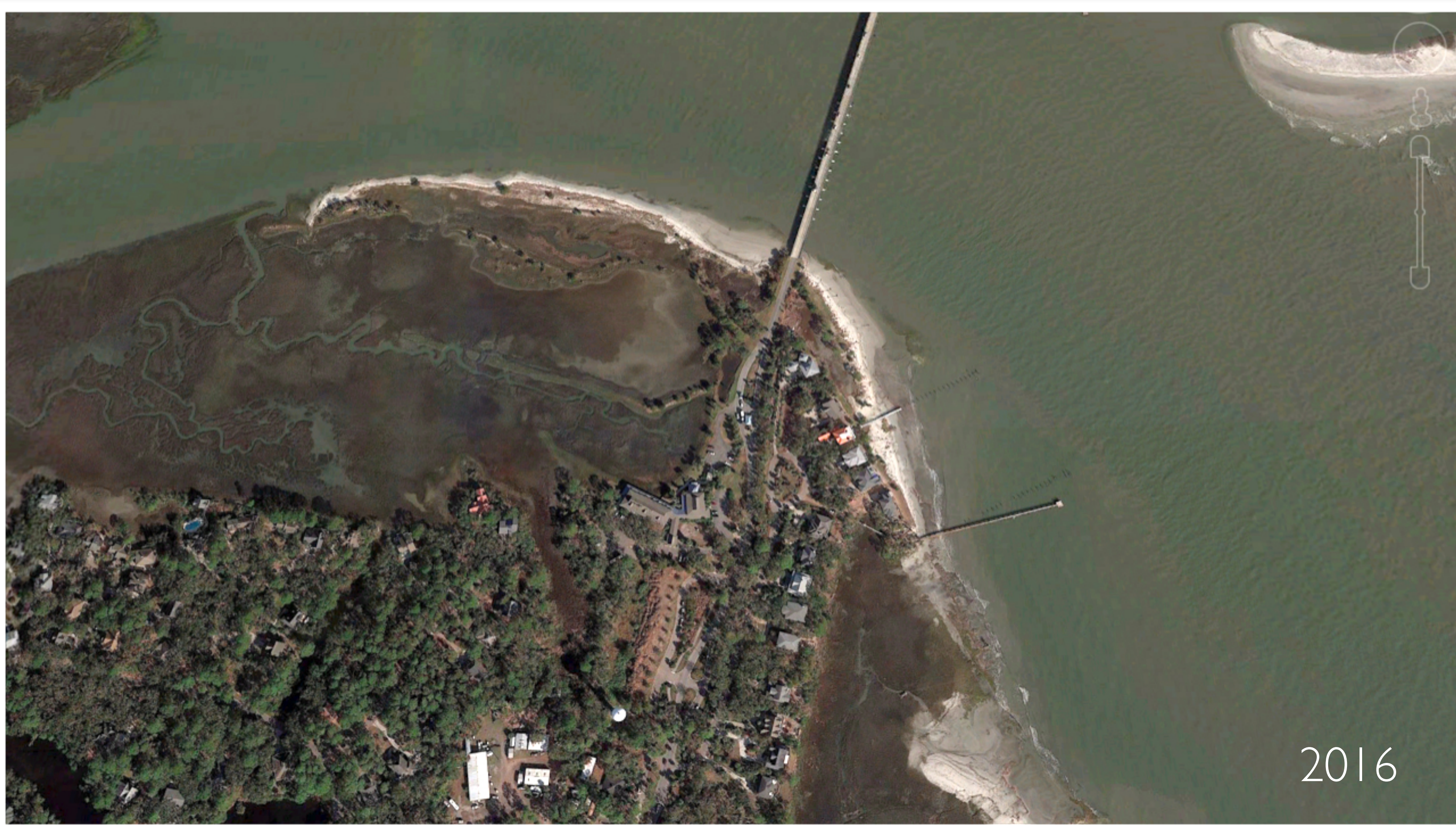
The bridge area of Fripp Island
