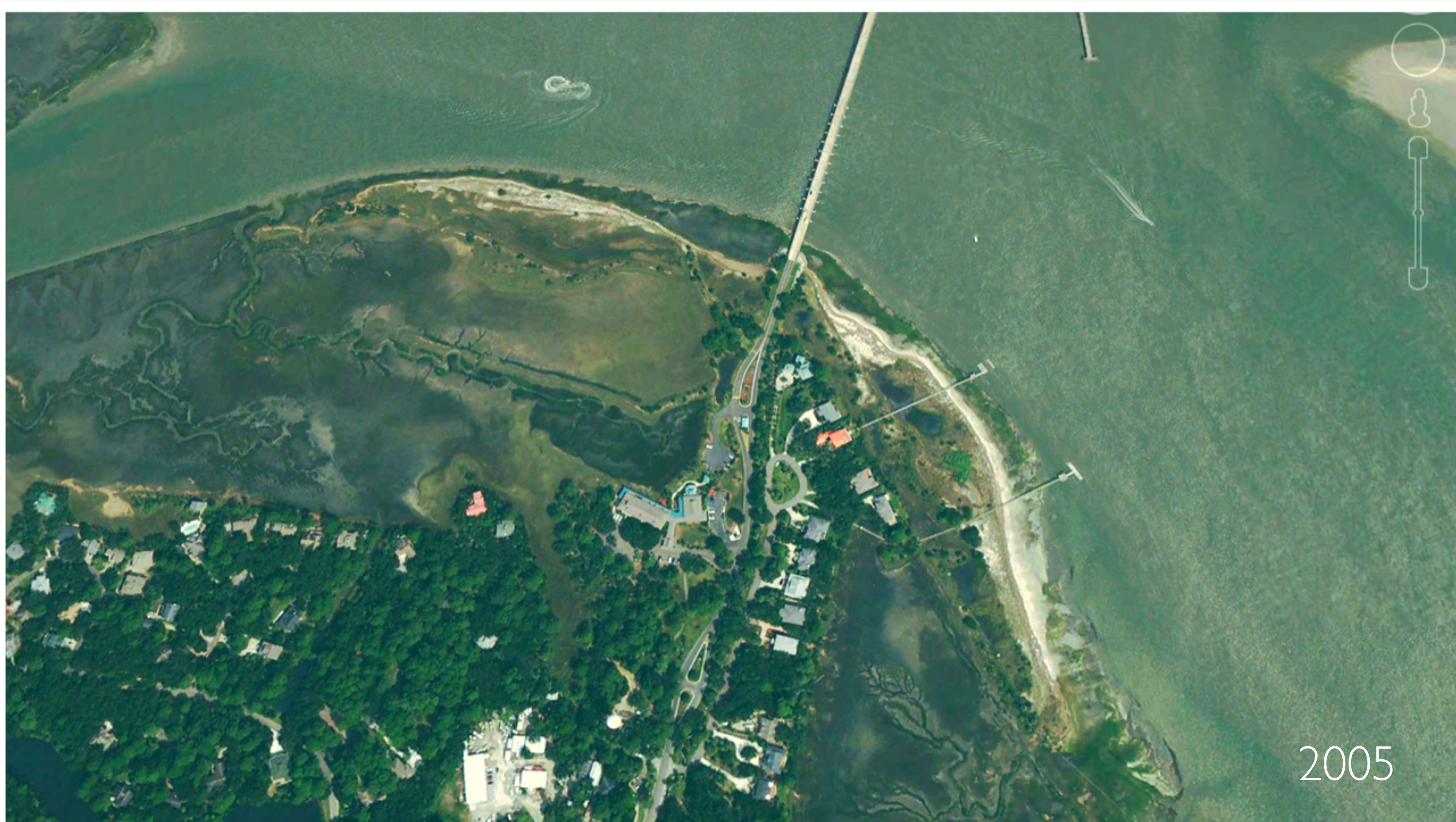
The bridge area of Fripp Island
